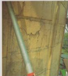
Detail of the plasterwork, highlighting how decayed the water tower was before renovation.
